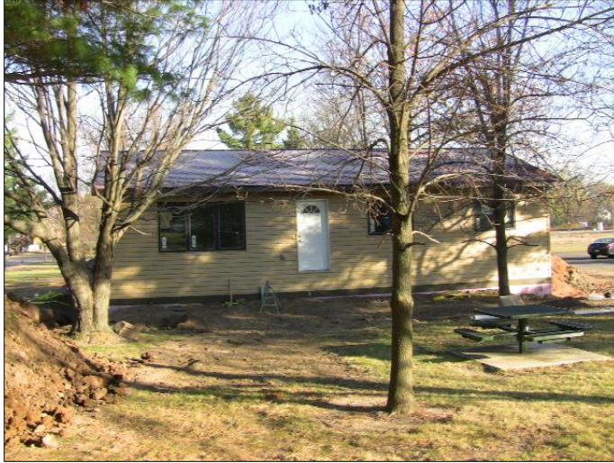
Photo above: The new house, built by students in Pine City High School's building trades course, is readied for occupancy at the northwest end of the campus.
